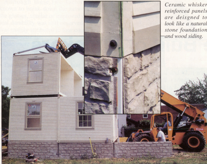
Prefabricated segments allow the house to be assembled in a few days.
