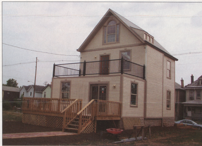
The exterior of the house is made entirely of the ceramic whisker reinforced resin composite, including the door and window frames, shutters, and roof.
